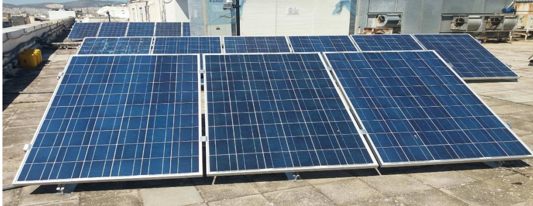
FIGURE 7: PART OF THE SOLAR PANELS INSTALLATION
